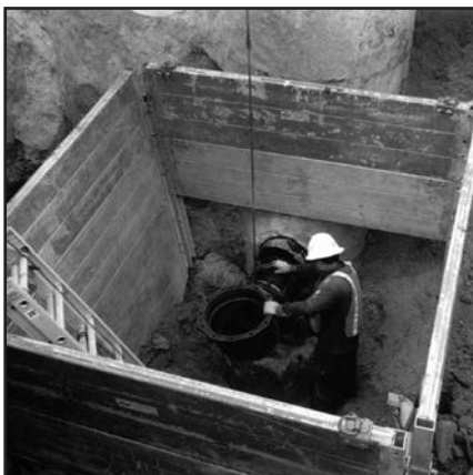
Four-sided configuration with sectional corner posts and removed bottom panel
