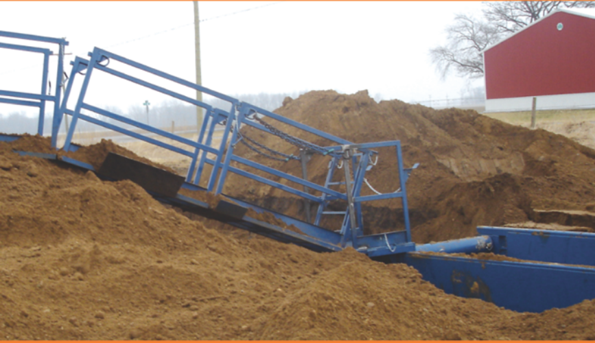
An assembled Walkway Bridge being moved into position at the jobsite.
